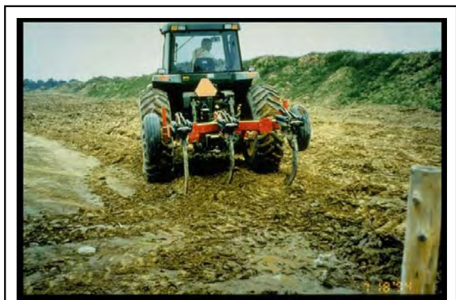
Fig. 9. This medium tractor is pulling a 3-shank deep ripper. The severely compacted construction access corridor is narrow, and the 120 hp tractor is more maneuverable for Phase 1 deep ripping (subsoil fracturing), here.
