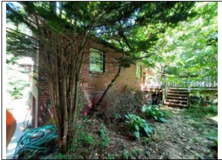
32. View of 475 Beaver Dam Road – Exterior
