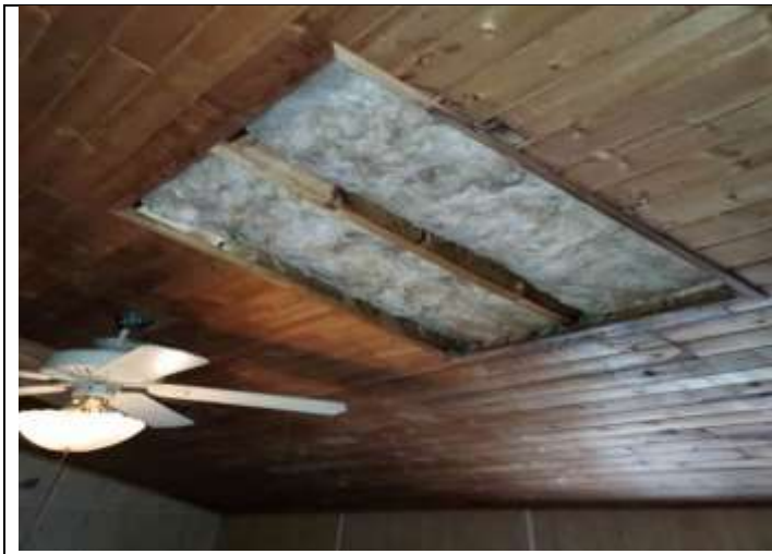
27. View of 497 Beaver Dam Road – Fiberglass Ceiling Insulation
