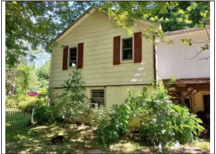
20. View of 497 Beaver Dam Road - Exterior
