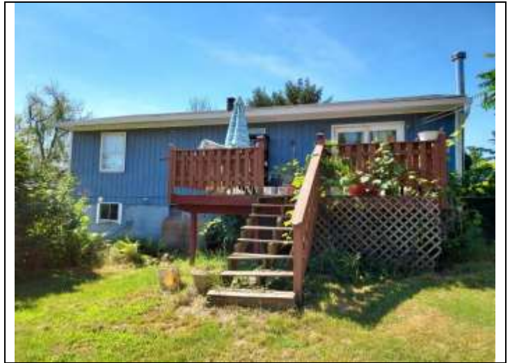
2. View of 355 Neelytown Road - Exterior Rear
