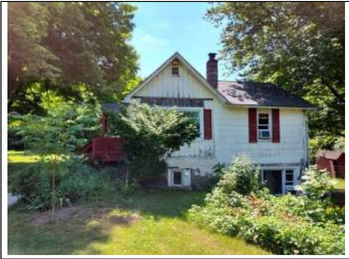
19. View of 459 Beaver Dam Road - Exterior
