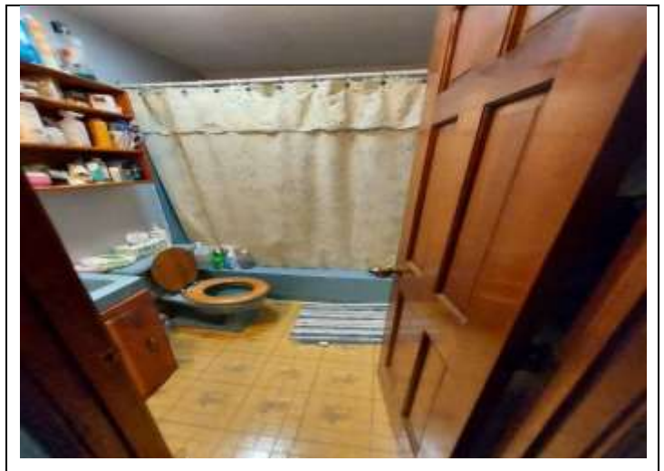
6. View of 355 Neelytown Road - Bathroom ACM Linoleum
