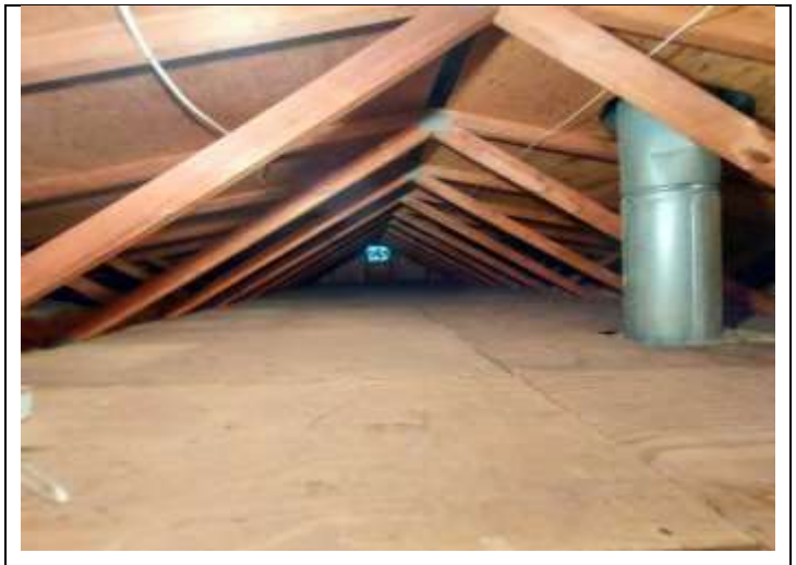
18. View of 497 Beaver Dam Road - Attic
