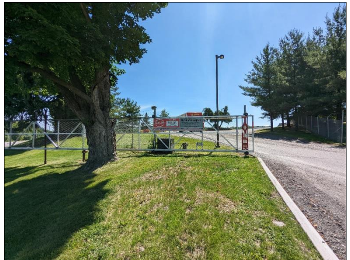
22. South adjoining recycling facility
