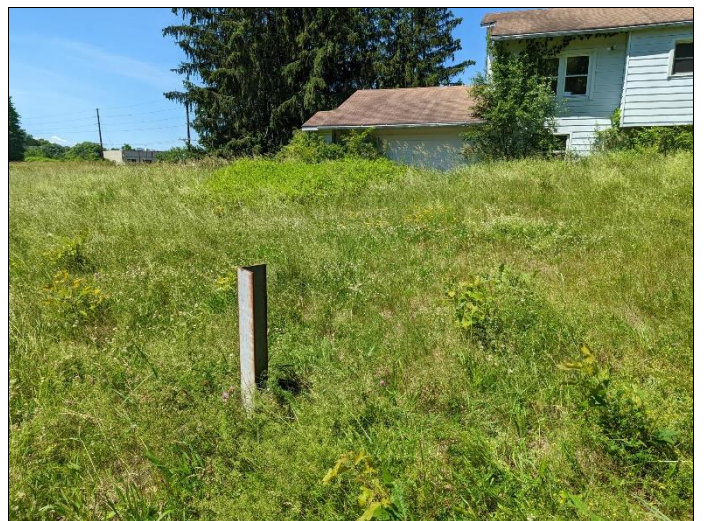
12. Well head structure on 483 Beaver Dam Road
