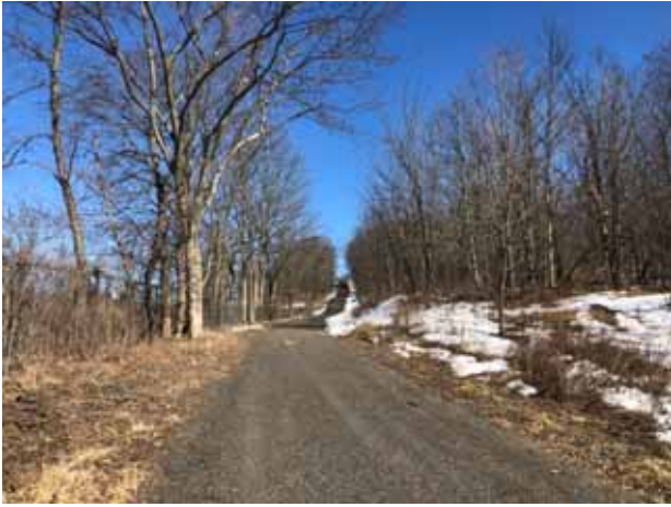
7. Service road looking northeast
