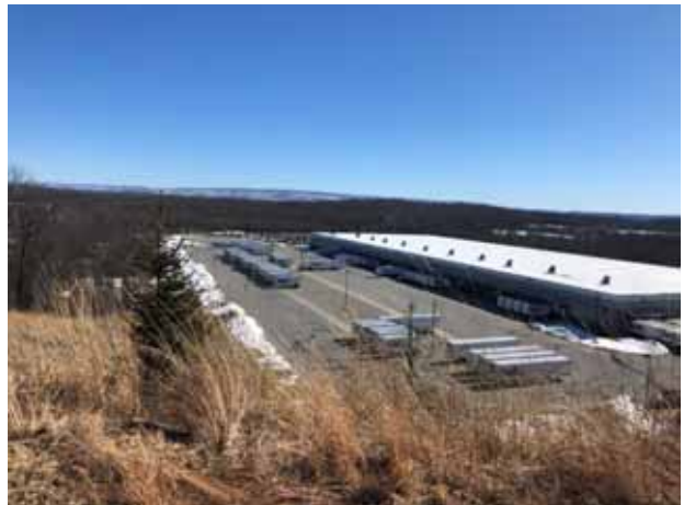
24. Southeastern adjacent Fedex Ground Trucking Terminal
