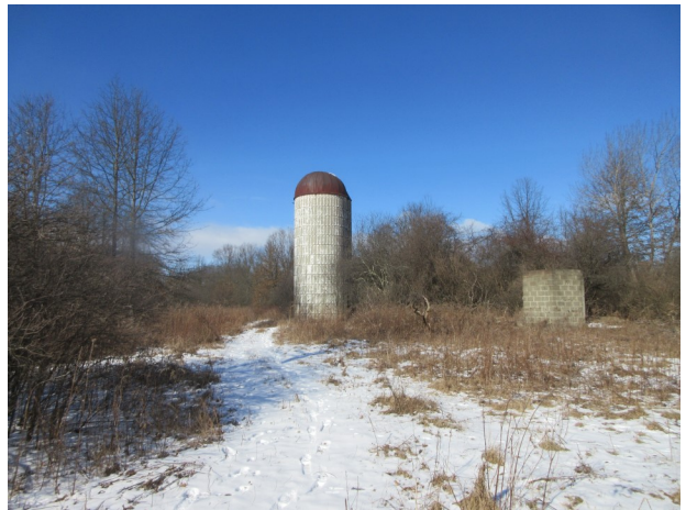
10. View of silo and masonry structure chimney remnants
