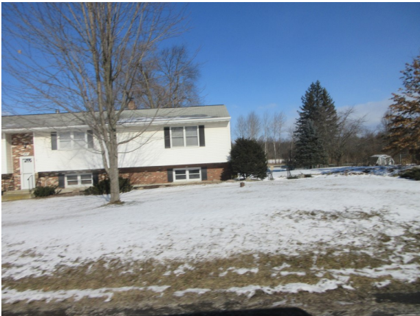
23. View of southern adjacent property
