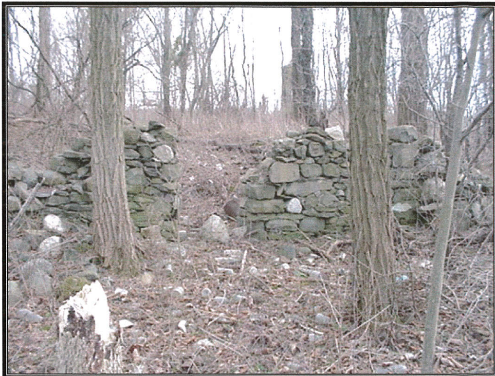
Figure 14: Site photo # 5 showing 2nd foundation ruins view east - BTK 12/04
