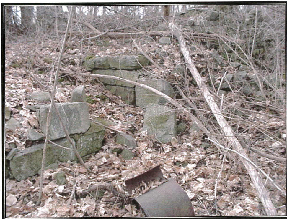
Figure 12: Site Photo # 3 showing part the Van Alst Foundation
