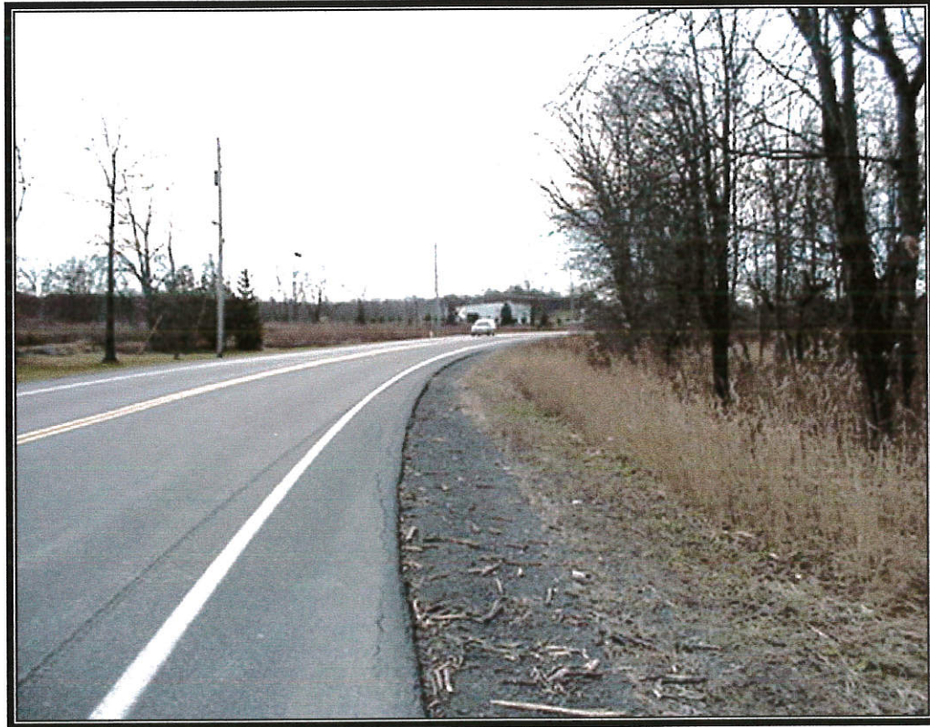
Figure 10: Road View South on Neelytown Road Photo # 2
