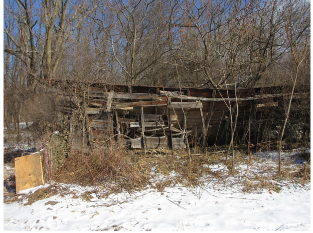
8. View of abandoned wood debris
