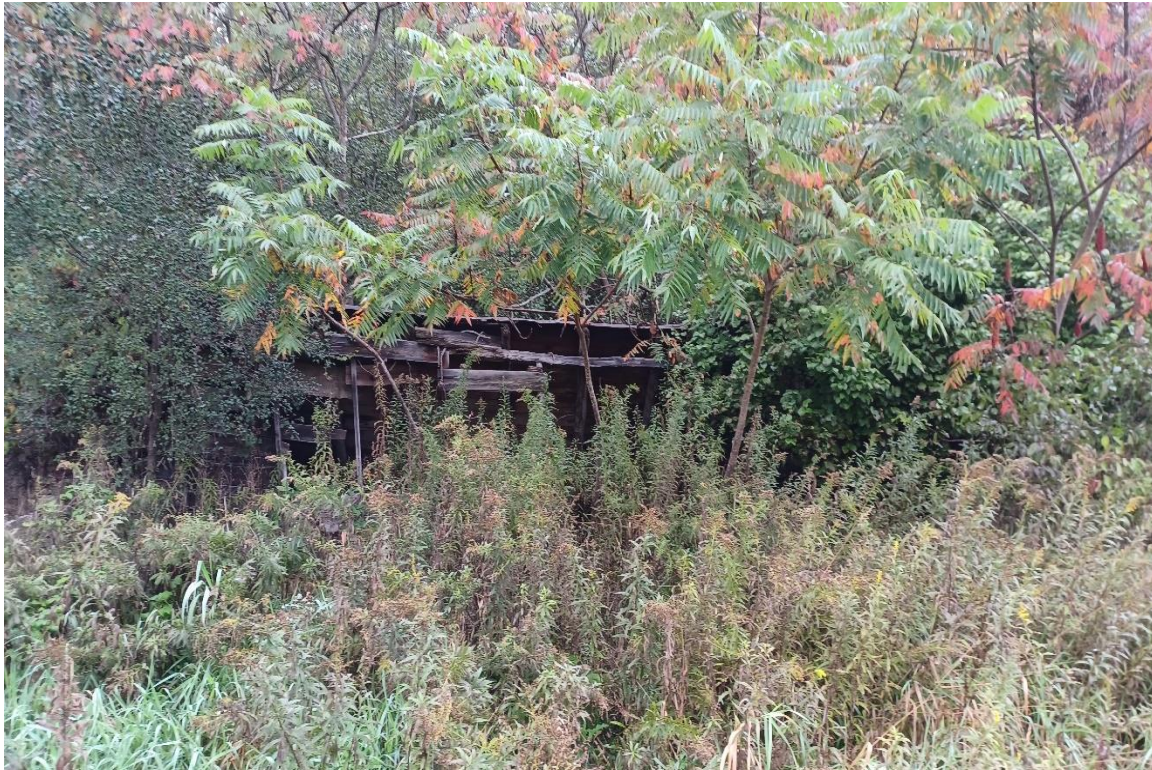
Photo 4: A wooded barn (F3) is located in the southeastern portion of the APE, south of the stone foundation. View to the north.
