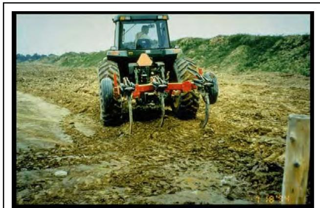
Fig. 9. This medium tractor is pulling a 3-shank deep ripper. The severely compacted construction access corridor is narrow, and the 120 hp tractor is more maneuverable for Phase 1 deep ripping (subsoil fracturing), here.
