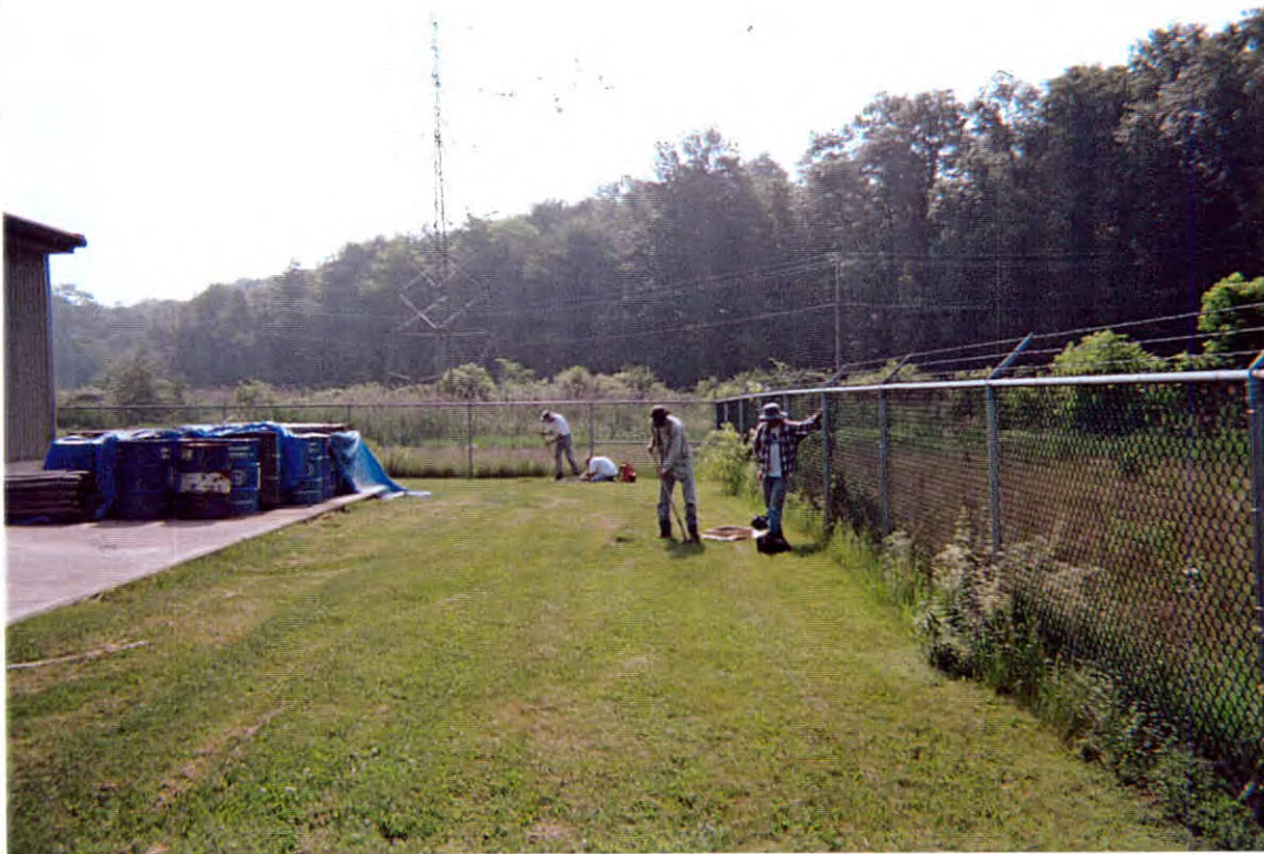
Figure 1.15 Water Line Route Sewer Plant Looking East.
