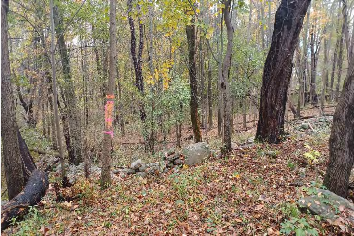
Photo 8: The southern boundary is defined by a stone retaining wall. View to the south.
