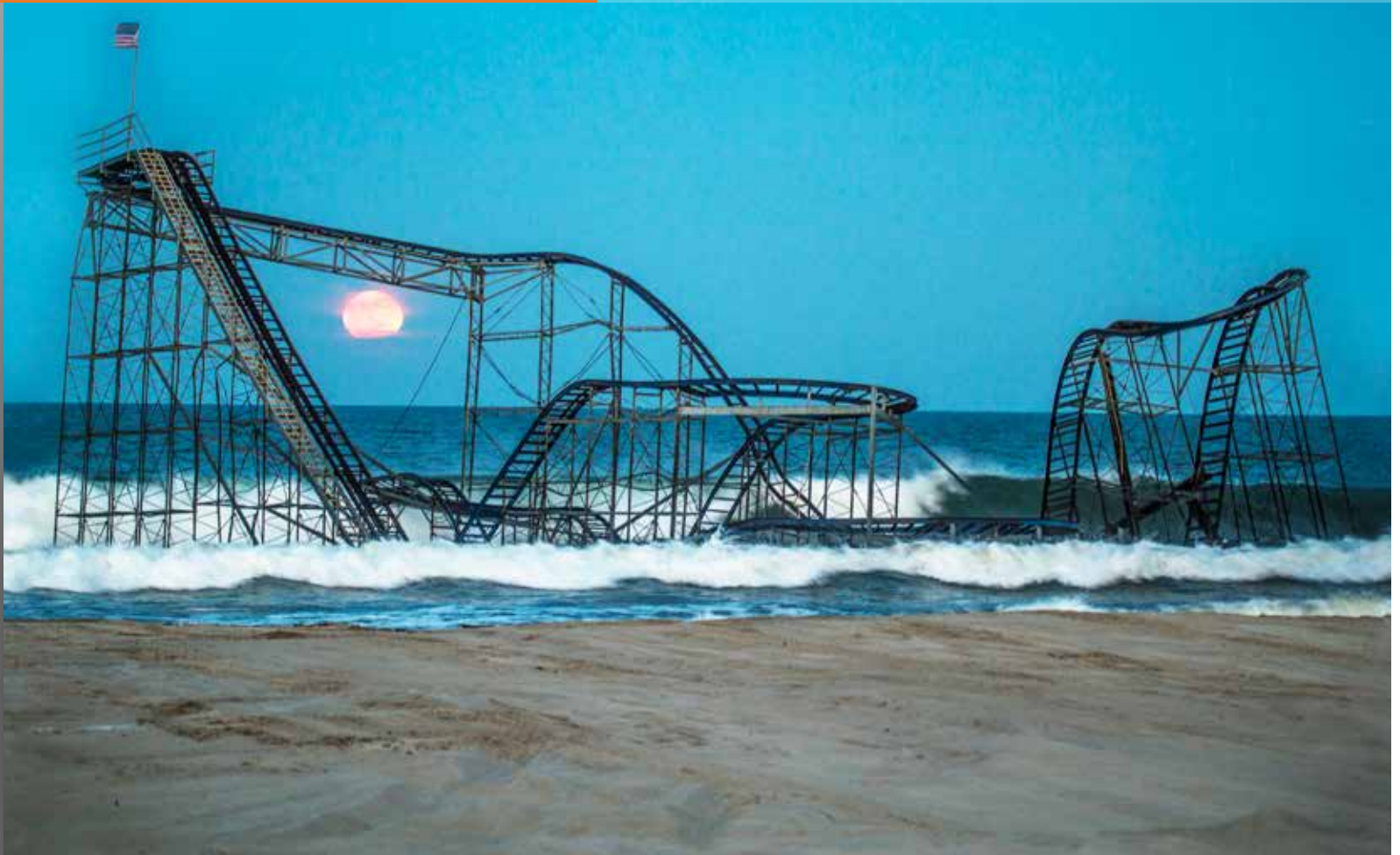
SuperStorm Sandy destroyed the Casino Pier in Seaside Heights, N.J., and left the Jet Star roller coaster stranded offshore. Before construction of the new pier could begin, the Jet Star had to be dismantled. Photo: Chris Spiegel Blurrevision.com
