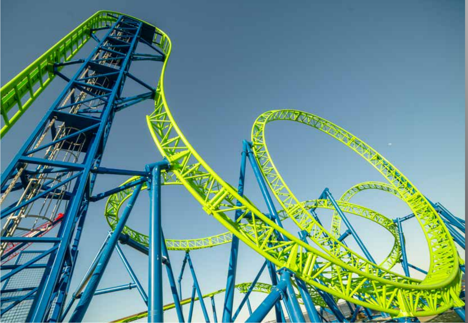
Lift tower foundation reactions exceeded 50 tons of uplift and downward forces resulting from the 72-foot-tall tower's ocean wind exposure and narrow base. The tower required a foundation unique from the rest of the coaster. Photo: Chris Spiegel Blurrevision.com
