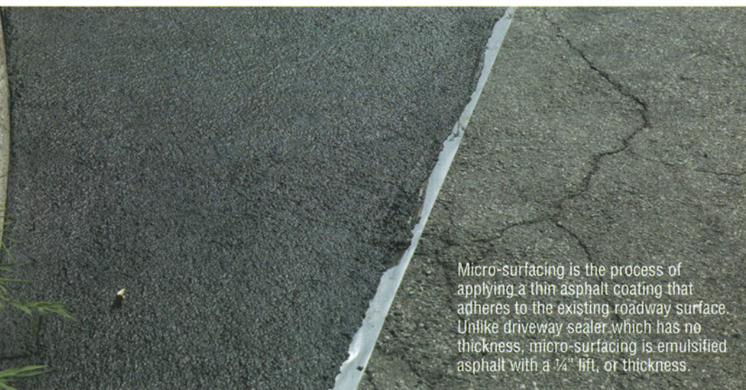
Micro-surfacing application begins after roadway sweeping.
