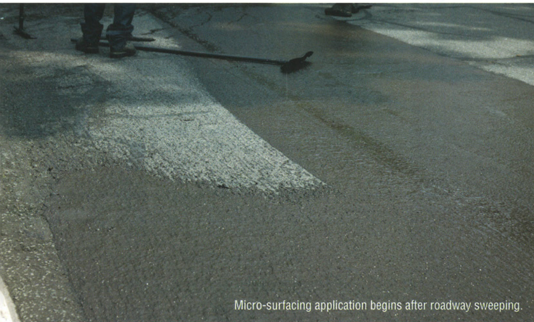
Micro-surface asphalt slurry being applied
