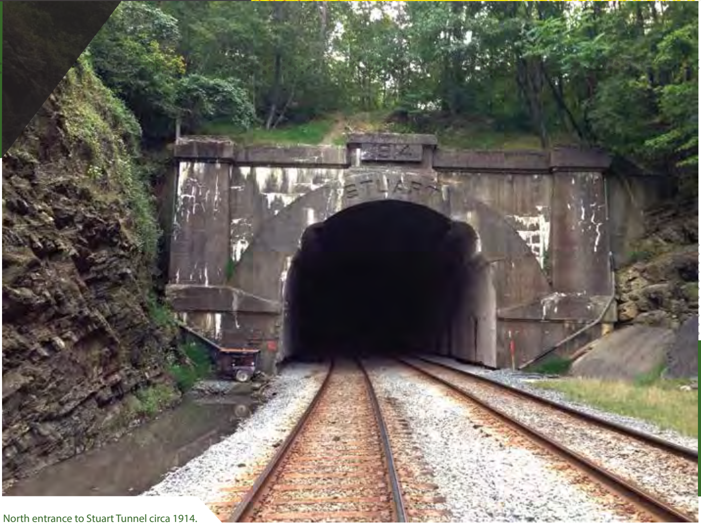
North entrance to Stuart Tunnel circa 1914.
