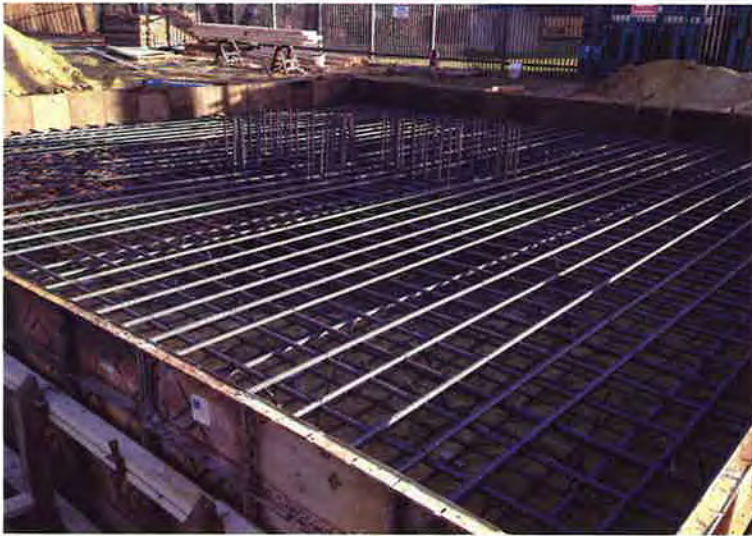
What the riders don't see: A footing under construction with multiple layers of steel reinforcement placed prior to receiving 24 trucks worth of concrete.
