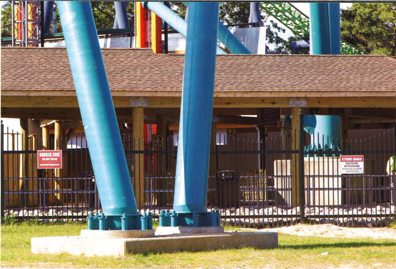
Like the tip of an iceberg, all that can be seen of the foundation system is the top of the shared concrete pedestal that provides support to two of the newly added support columns. Hidden below the surface is a 36-foot by 36-foot by 5-foot-thick concrete footing.
